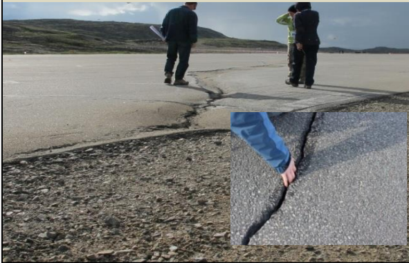
Frost cracks
